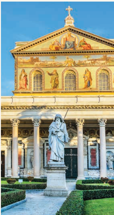
ST. PAUL'S OUTSIDE-THE-WALLS, ROME
